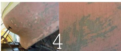
The second coat, a fairing compound, is plastered over the hull with a little less finesse, but then carefully sanded away to a smooth finish, restoring the hull's shape.
